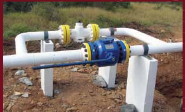
6" 600 ANSI Receiving valve, with full 6 inch bypass.
